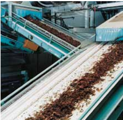
Inclined conveying in the tobacco industry. In this area, conveying angles of up to 22° are possible for belt types with smooth surfaces.
