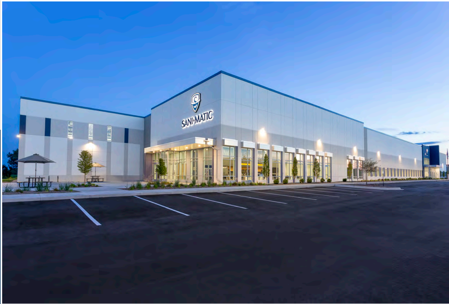
Components fabrication and distribution comes out of our primary manufacturing facility in Sun Prairie, WI, USA
