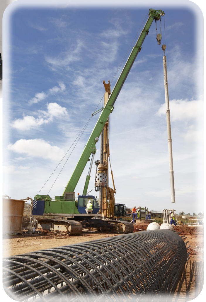
Crawler Telescopic boom Crane
