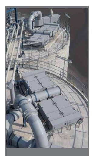
A compact design with numerous geometric variants and different lengths of filter pockets permits the optimum adaption to procedural and spatial situations.
