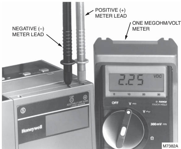
Fig. 11. Measuring flame signal voltage of 7800 SERIES controls.
